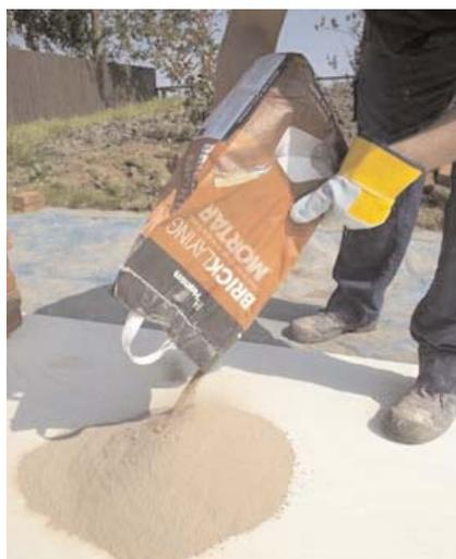
Ready mixed dry mortar is produced in 25kg bags and where these are stored on site it is essential that they are covered and stored in a dry environment. Bags should also be used in rotation and care taken to comply with the usage dates printed on each.
