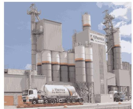
Dry mortar is also ready-to-use, with the exception of the mixing water which is added on the construction site. Production utilises similar plant to that for wet mortar although the units are invariably much more sophisticated. They generally incorporate a fine aggregate (sand) drier, although this is not essential if the aggregate feedstock has been pre-dried.
