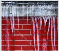
If the temperature of recently laid mortar falls below 0°C there is a probability of some degree of frost attack. The water may freeze and expand thus disrupting the mortar by forcing the material apart and breaking the bond.
