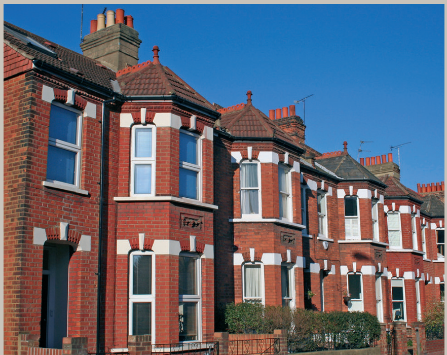
Twenty-five per cent of UK housing stock is of solid nine-inch brick construction.
