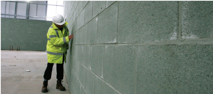
Assessing the green mortar at the new sports complex
