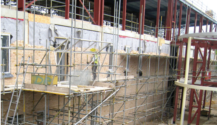
Brickwork and blockwork well underway at Lister Hospital
