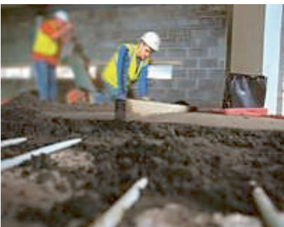
Laying a cementitious floor screed
