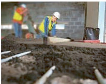
Laying a cementitious floor screed
