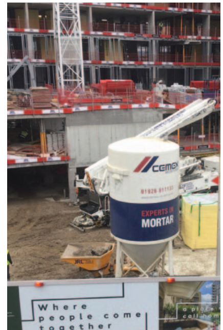
CEMEX dry mortar silo at the Wembley Park construction site
