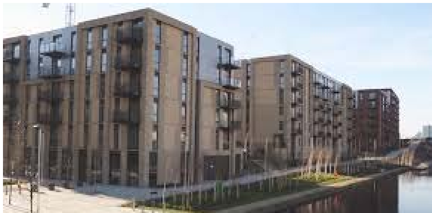
Middlewood Locks development.
