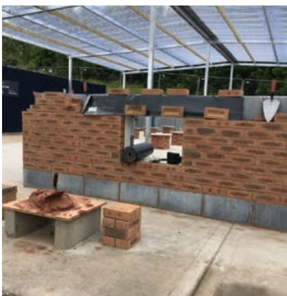
The covered area for practical work.
