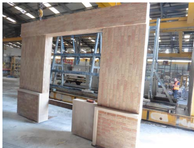
Finished brick panel at the factory.
