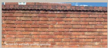
A data sheet, 'Repointing external brickwork', explains that mortar in poor condition can lead to a loss in wall strength. This is often found in old properties where mortar is powdery or easily scraped away so that the joints are appreciably recessed. Incorrect use of pressure cleaning of fresh mortar in new masonry can also affect the strength of new construction and must be avoided.
