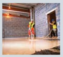
The type of screeding mortar used will depend on the required strength and end use. Levelling screeds are designed for a number of applications and to receive a final flooring, the thickness of the screed is governed by the method of construction being used. To achieve the optimum performance from a levelling screed a high standard of workmanship is essential.
